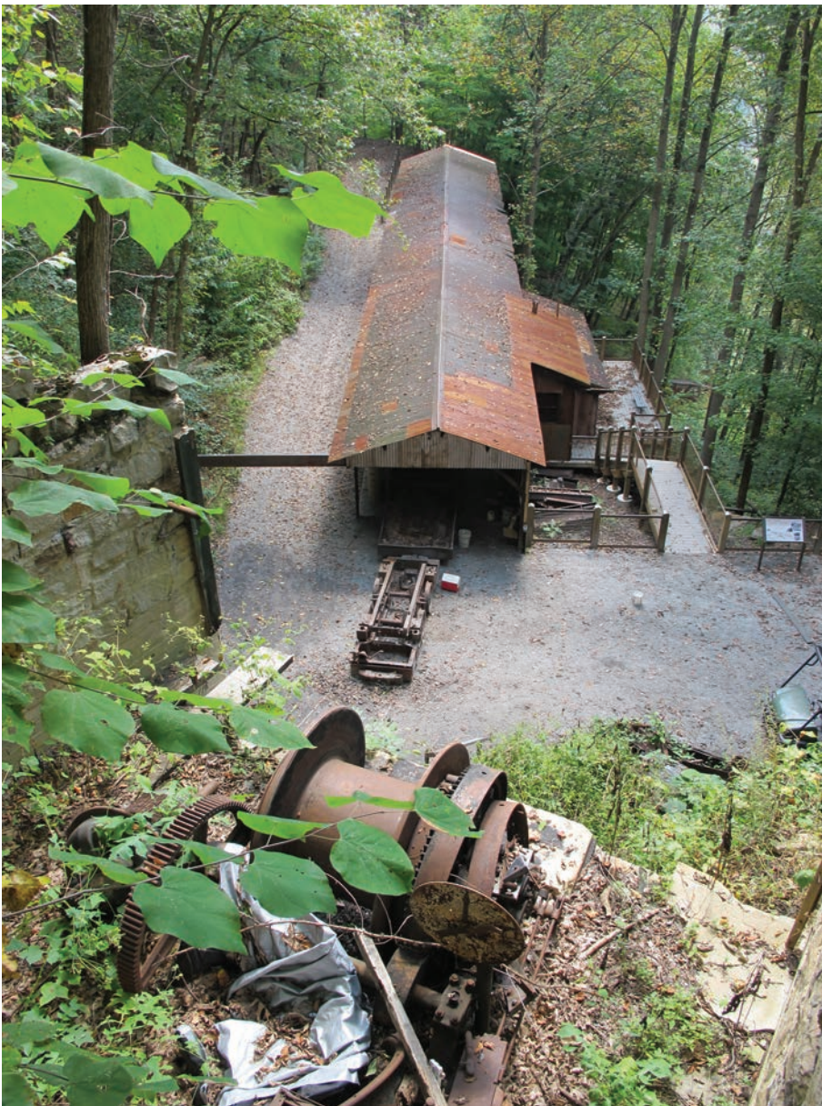
Overhead view of the headhouse, where coal was weighed and loaded onto the conveyor
