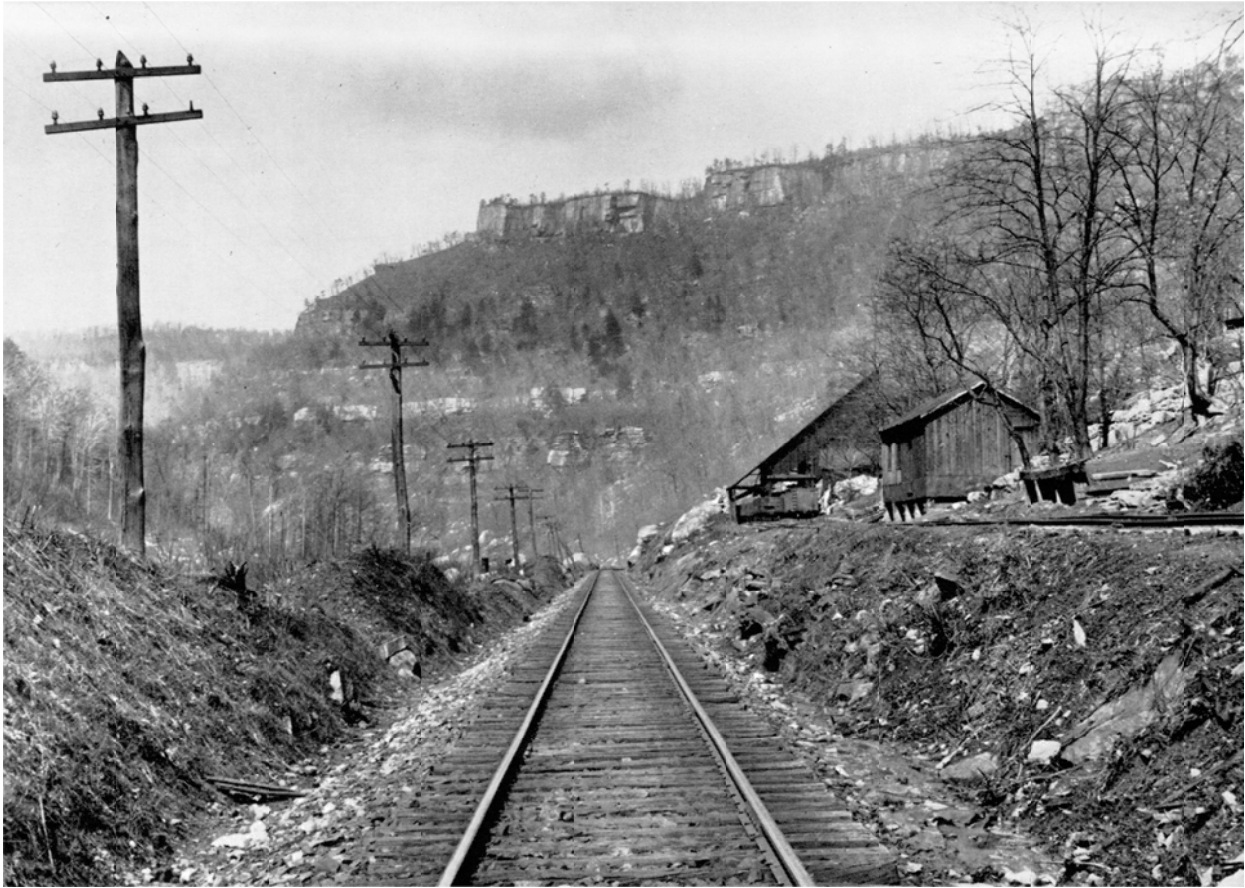
Photograph 9 – 150 Feet Below Nuttall Station
