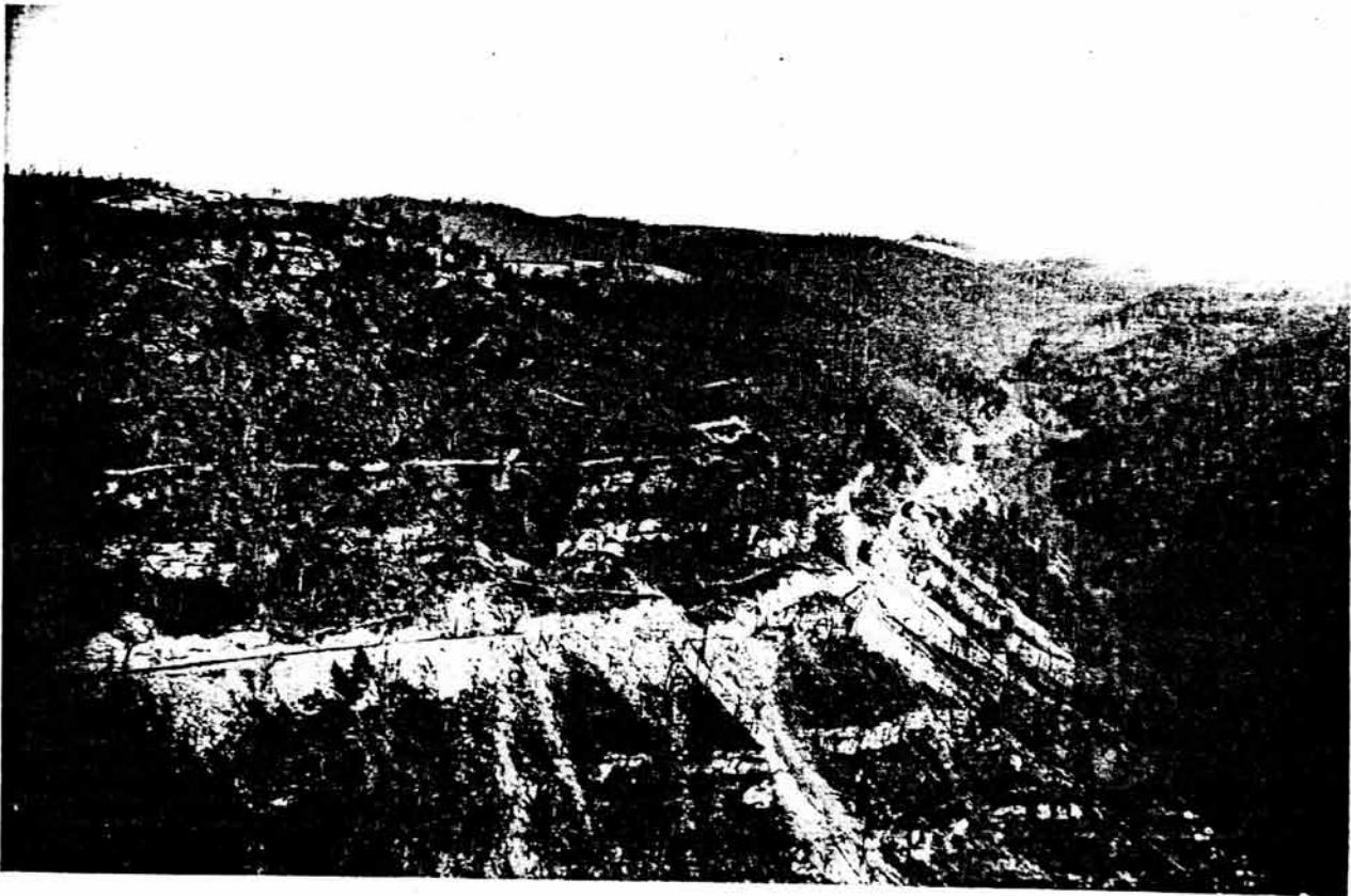
CONSTRUCTION — KEENEY'S CREEK R.R.
