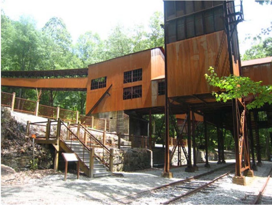
Restored tippel and conveyor
