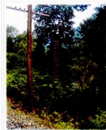
Remains of suspension bridge at Nuttallburg that once linked the two mining towns on opposite sides of the New River
