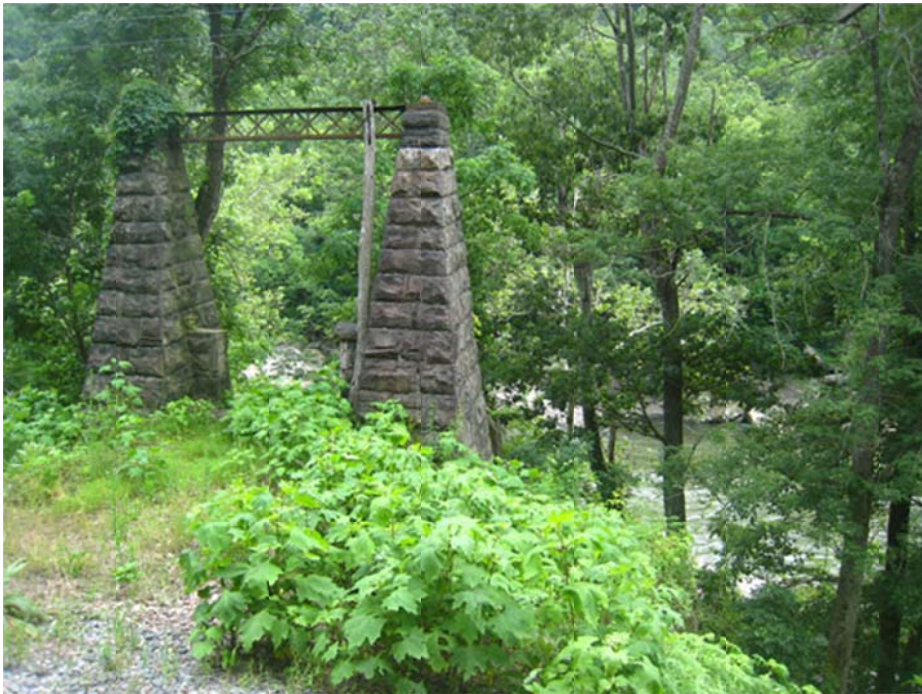
Piers that supported suspension pedestrian bridge that crossed the New River and connected Nuttallburg with South Nuttall (sometimes called Brown). Interestingly, the bridge was built by the Roebling Co - the same co that built the Brooklyn Bridge.
